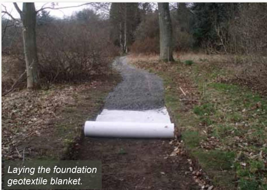
*Laying the foundation geotextile blanket.*
