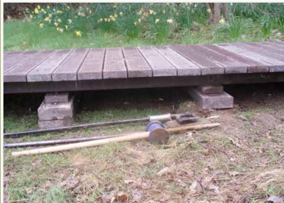
*Boardwalks can be supported on driven posts or bearers that lie on the ground. Either way, water can flow past freely.*
