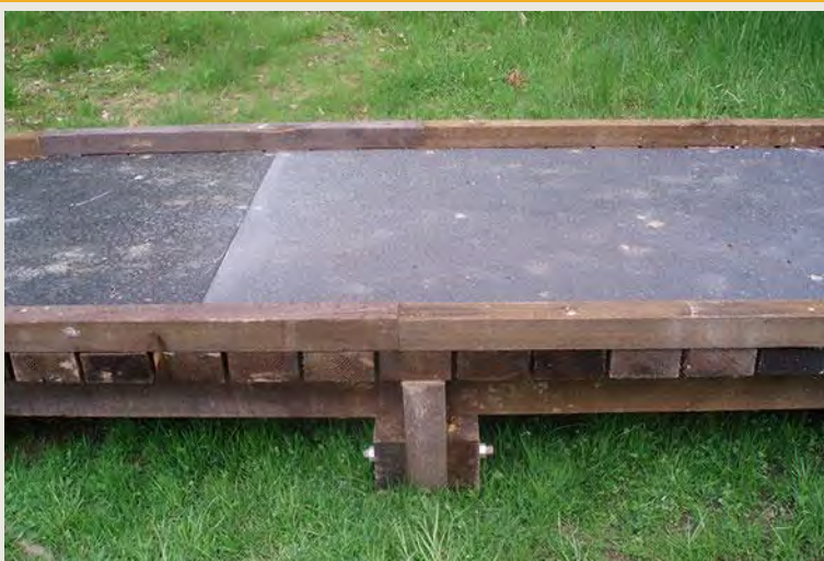
Timber boardwalk with a plastic stob
